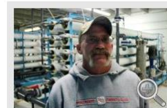
Creighton, Nebraska water operator, Kevin Sonnichsen, stands before the $1.3
