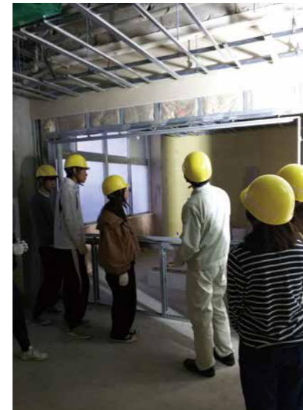
Observation of the building during construction
