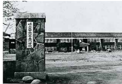
Unuma Temporary School Building (1963)
